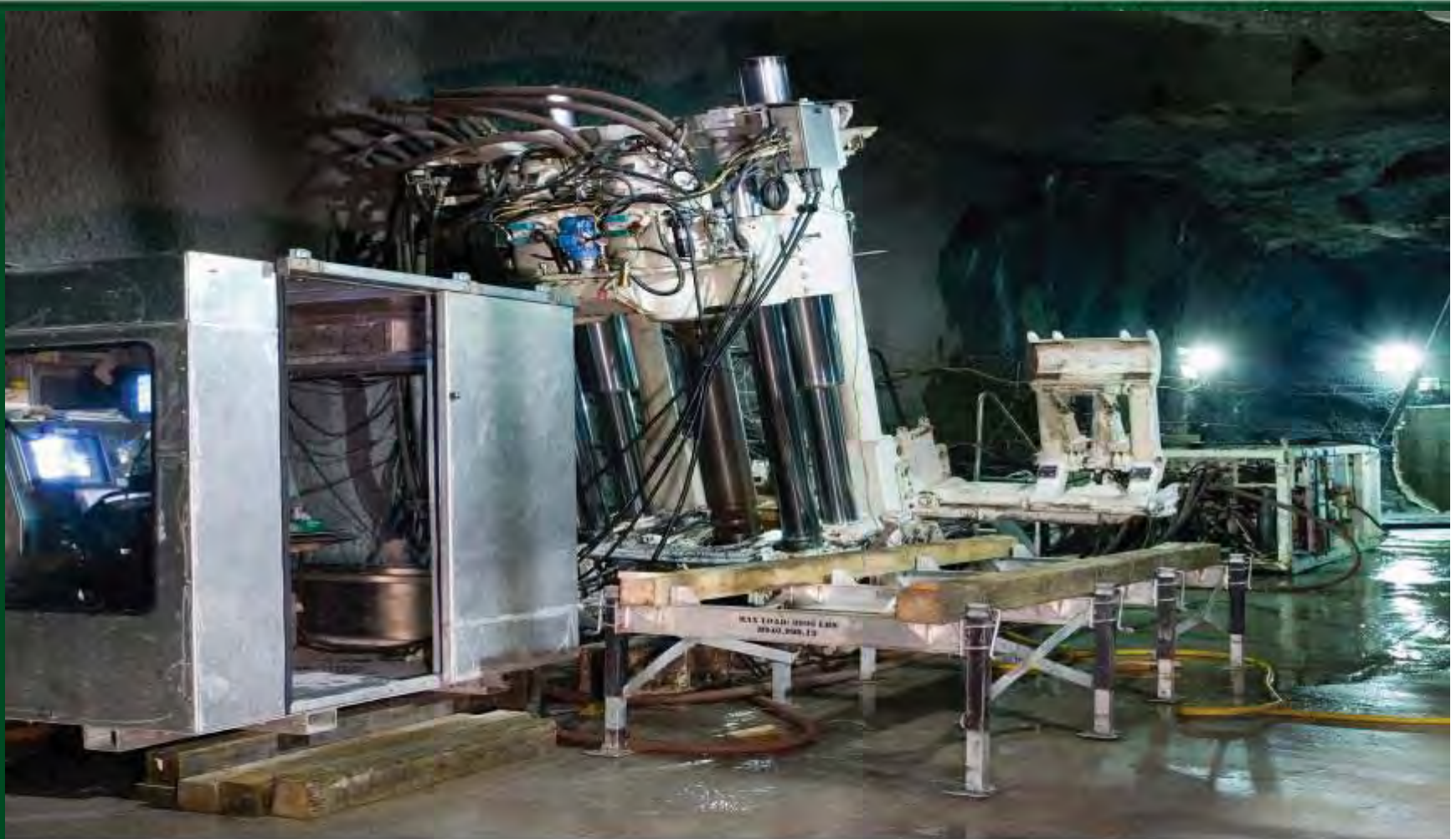
Raisebore Drilling at McArthur River From the 530 metre level a pilot hole is drilled down through the ore zone into the tunnel on the 640 metre level.
