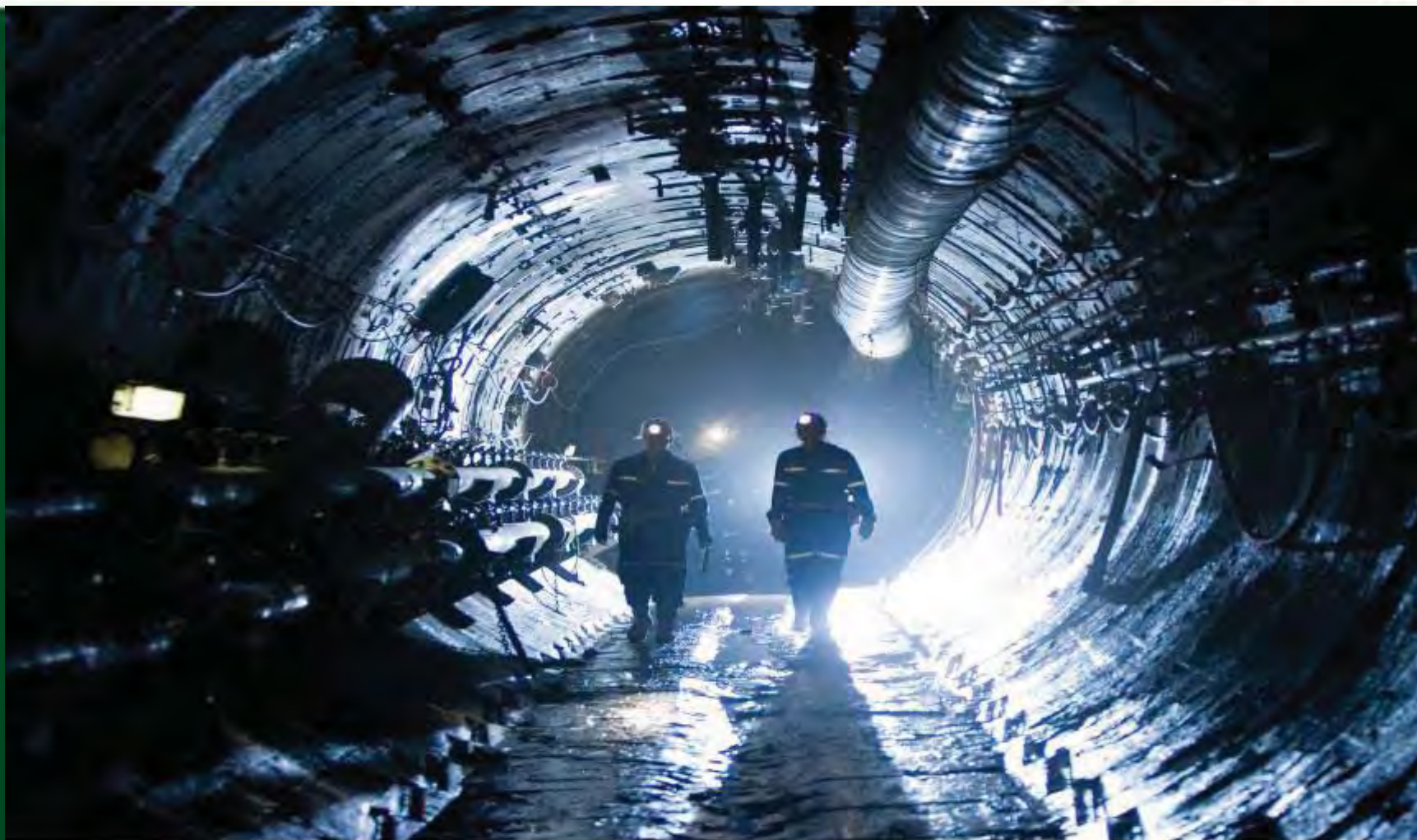
Cigar Lake Underground tunnels at Cigar Lake are reinforced with concrete to ensure a safe working environment.
