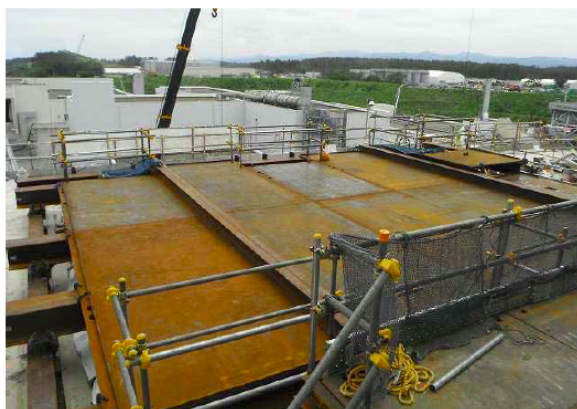
Protection platform installation on the Spent Fuel Pool Photo taken on June 15, 2012
