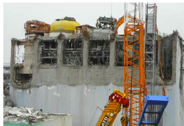
After debris removal (Upper part of the operating floor, west surface) Photo taken on July 9, 2012
