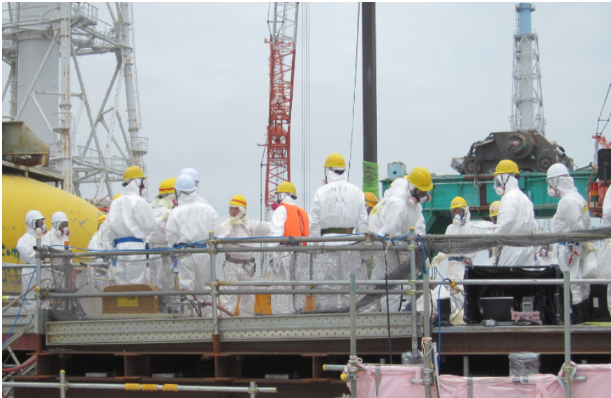
Figure 29: Unused fuel bundle being lifted out of the Unit 4 Spent Fuel Pool
